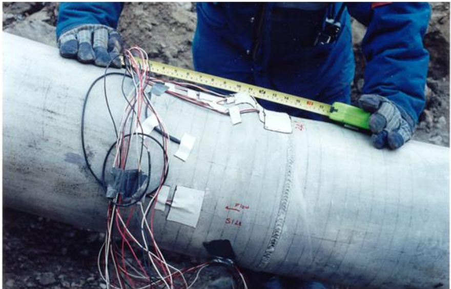
Figure 4.4 Wrinkle formed in NPS 12 pipeline due to soil movements.
